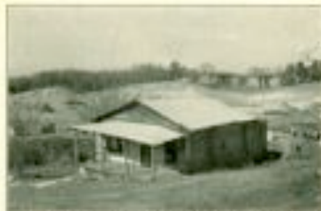
House Sited for Demolition, Oxford, Mississippi
