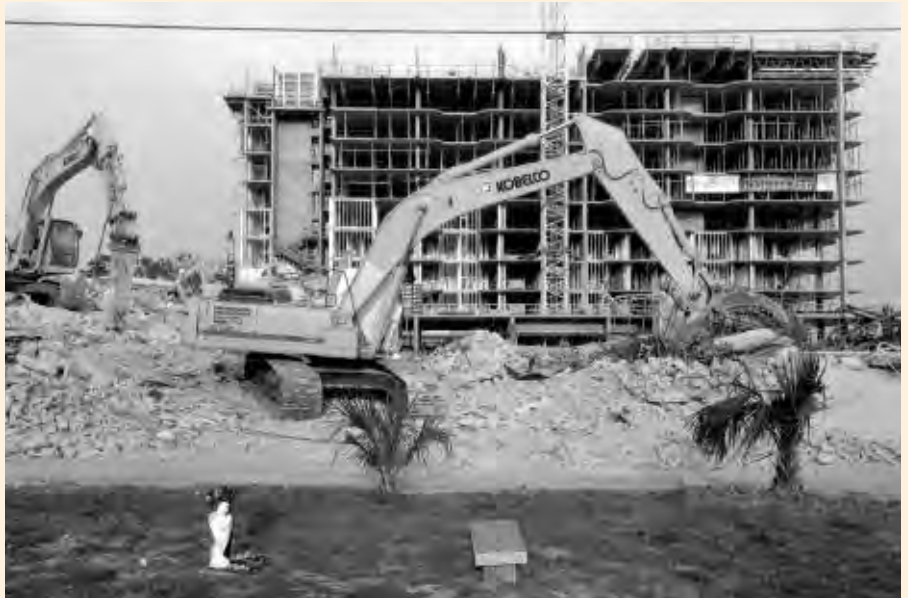
David Wharton: Construction Site by Cemetery, near Biloxi, Mississippi
