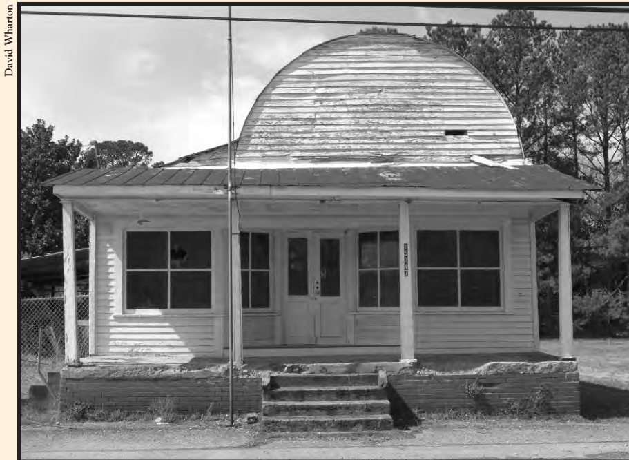
Abandoned building, Highway 411, Tennaga, Georgia
