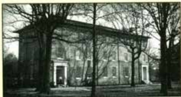
The Y Building
