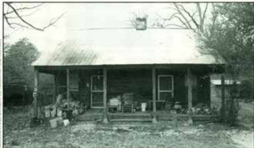
Saddlebag House: Robert Johnson House, Rankin County, Mississippi
